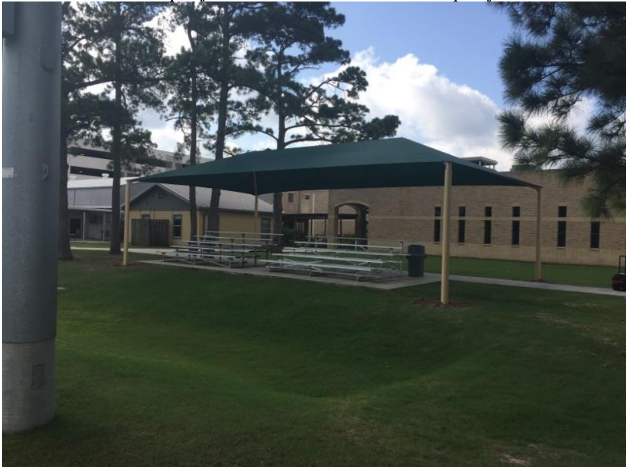
Example of Four column shade structure with hip roof
