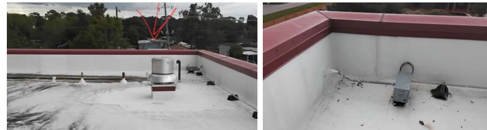
Backside @ rooftop parapet wall - For Reference
