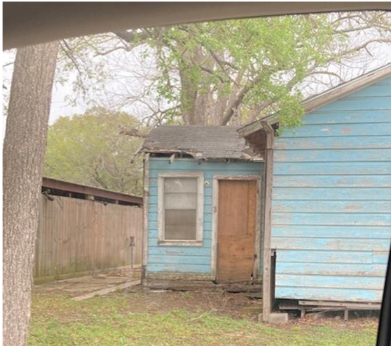
Holes in roof, rotted door frame, collapsed eaves
