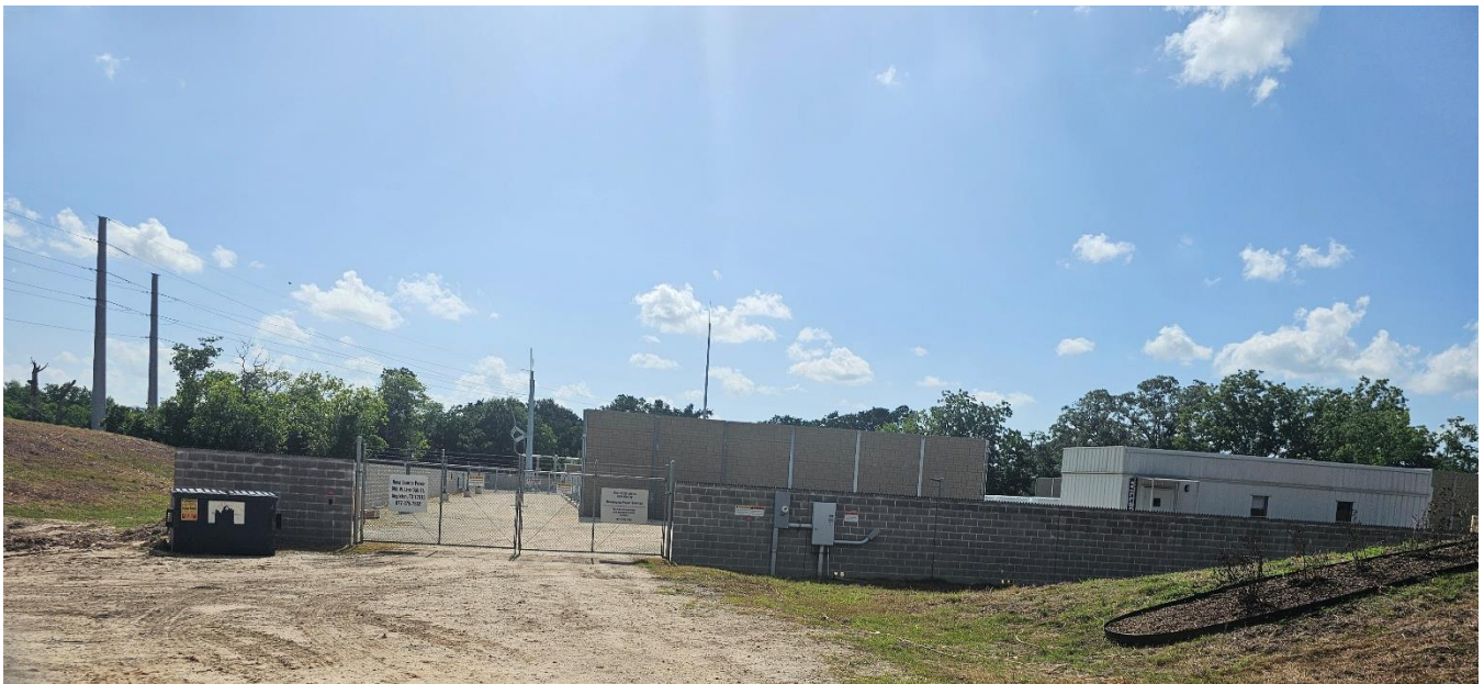
Photo of Sound Wall as Installed
