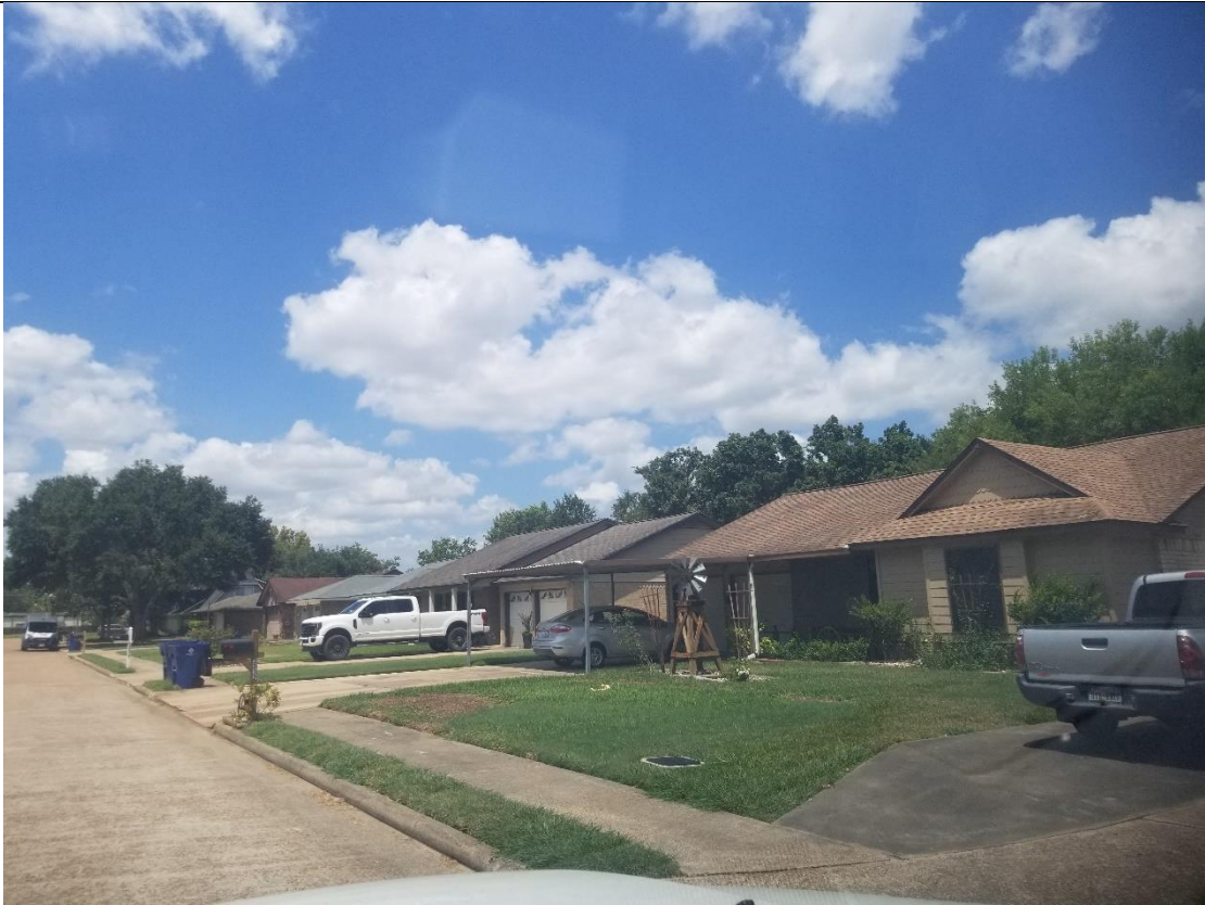
View of existing carport on diagonal rear lot
