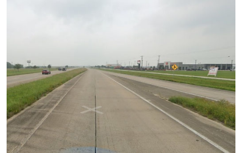
SH 288 Regional Corridor
