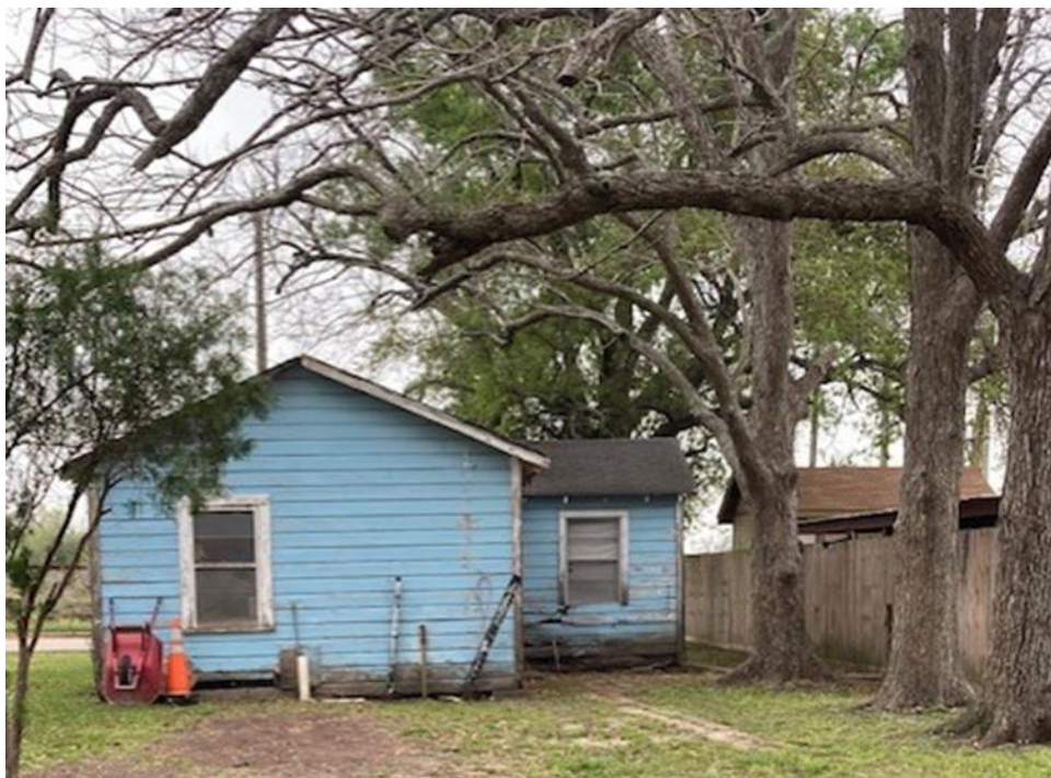
Rotted exterior siding, broken windows
