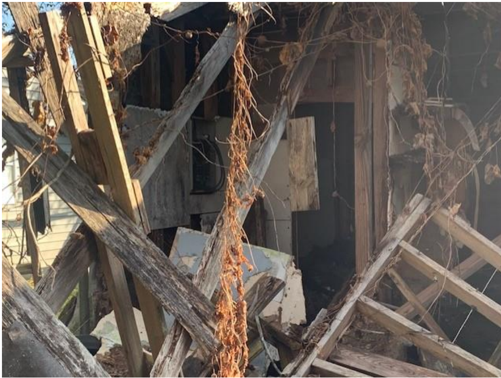
Backside of garage
