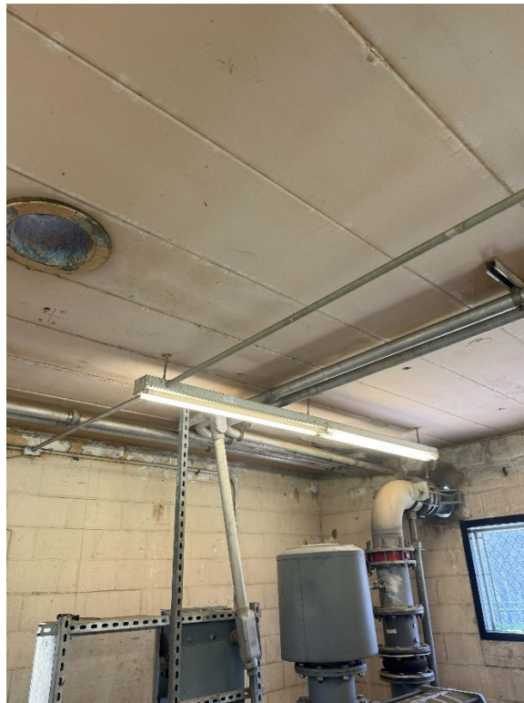
Figure 5 View of Blower Building ceiling and walls
