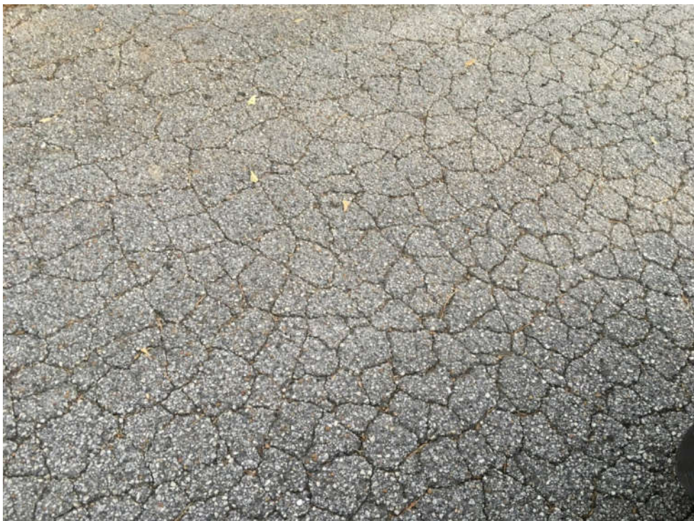
ALLIGATOR CRACKING
