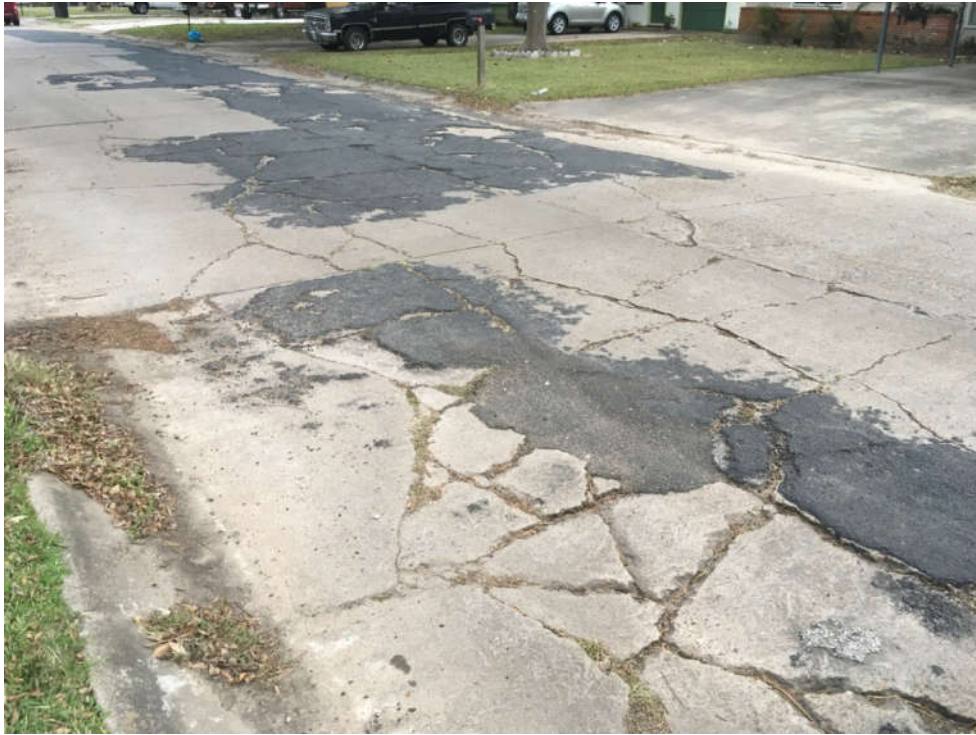
BLOCK CRACKING
