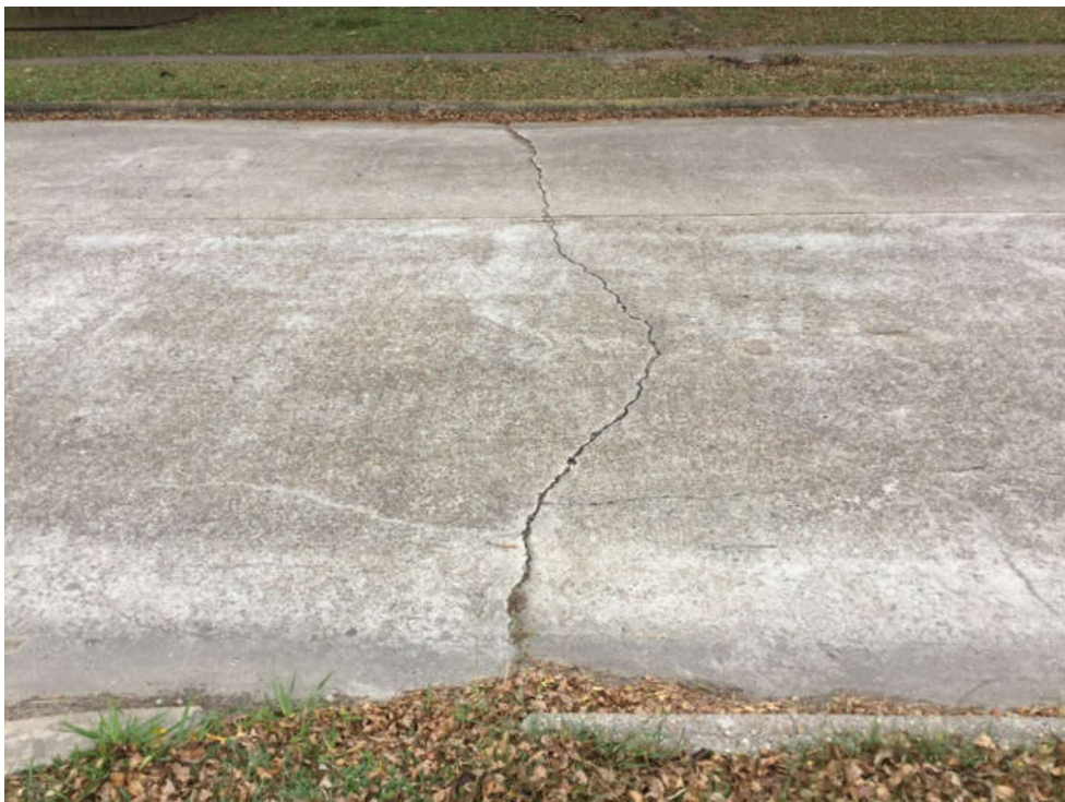
TRANSVERSE CRACKING
