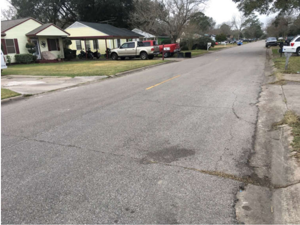
BLOCK CRACKING
