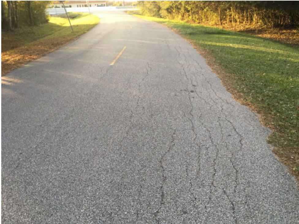
SLIPPAGE CRACKING
