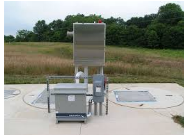
Typical Submersible Lift Station
