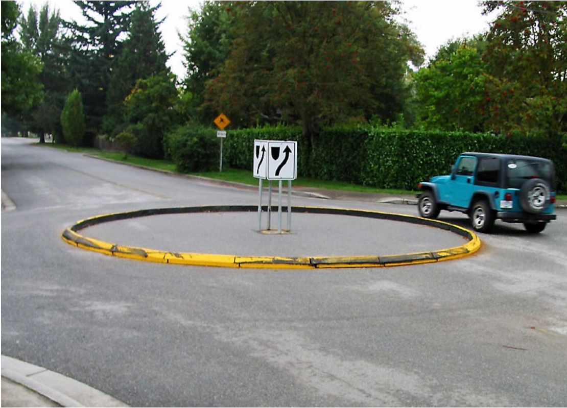
Figure 18. Example of a Temporary Roundabout Design
