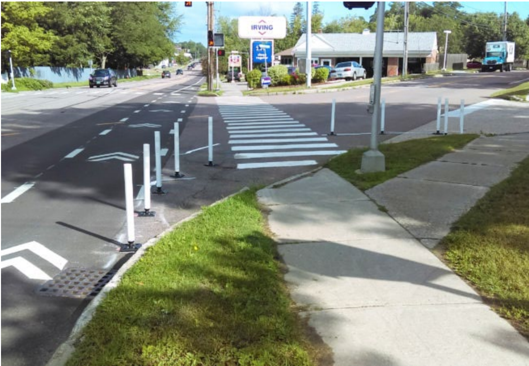
Figure 16. Example of Temporary Flexible Delineators
