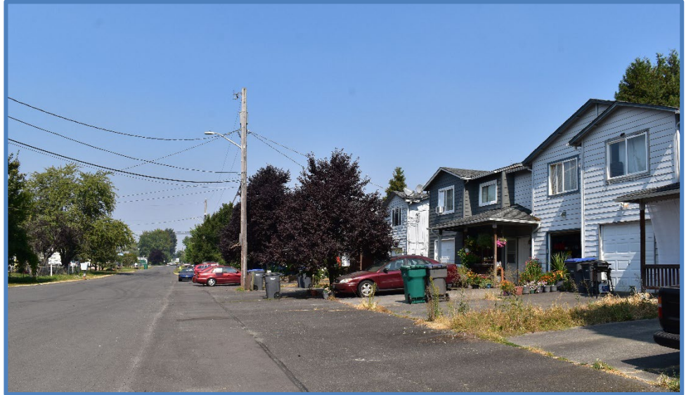
Above ground powerlines bring electricity to Algona's homes and businesses. The City is powered by Puget Sound Electric (PSE) who is responsible for system upgrades and billing rates. Photo by: Betty Padgett
