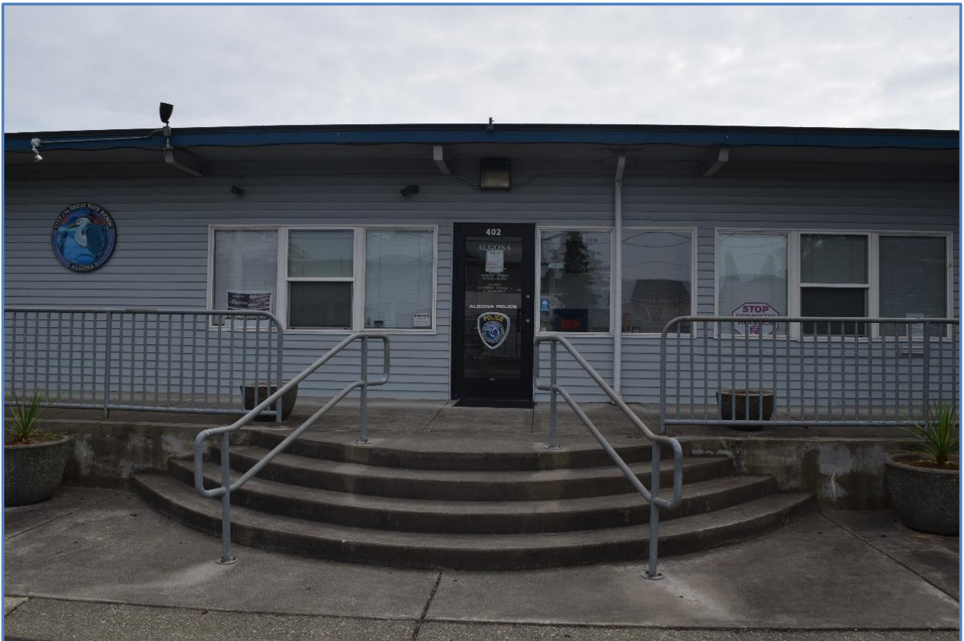
The City of Algona Police Station
