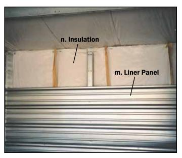
m. In insulated buildings, 29 gauge liner panel is used to cover the wall insulation and protect it from damage.
