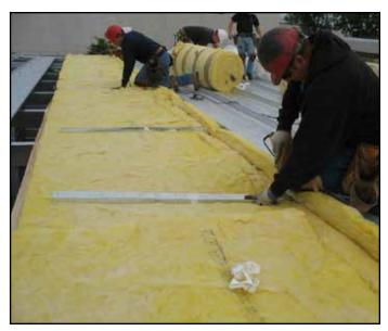
n. Trachte offers up to an R-38 (12") roof insulation. Shown above is a R-32 (10") roof insulation using R-5 thermal blocks. Contact a Trachte Regional Manager about meeting energy codes.
