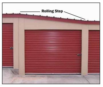
h. An alternate way to accommodate a roof step is to use a rolling step. This design can be used for steps up to 12" in height. Please contact the Trachte Regional Manager for limitations and other information.
