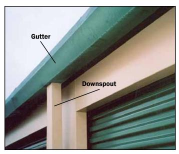
I. 26 gauge gutters and downspouts can match either the building or door color.
