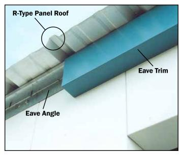
The screws at the eave are located outside the building to prevent roof leaks. The eave trim covers the eave angle and roof screws for a clean, finished look. This feature is standard on all Trachte buildings.
