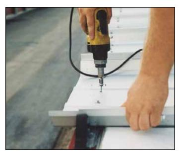
p. The standing seam roof need only be screwed down at the eave. This prevents having exposed screws across the roof sheets, minimizing the potential for roof leaks. Trachte highly recommends the standing seam roof, which features 2' wide snap together panels.
