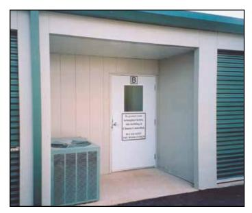
y. The 18 gauge flush recessed entry way is an ideal location for the HVAC unit. In addition, it gives customers a place to stage their goods during inclement weather.
