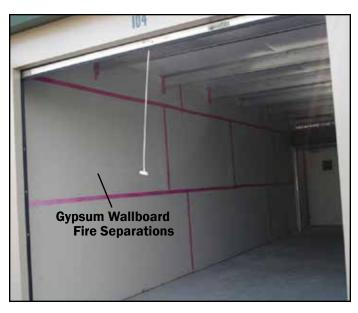
For interior fire separations, gypsum wallboard is installed over stud wall and taped. Number of sheets on each side of stud wall will vary based on fire rating needed.
