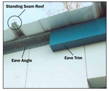
p. The screws at the eave are located outside the building to prevent roof leaks. The eave trim covers the eave angle and roof screws for a clean, finished look. This feature is standard on all Trachte buildings.
