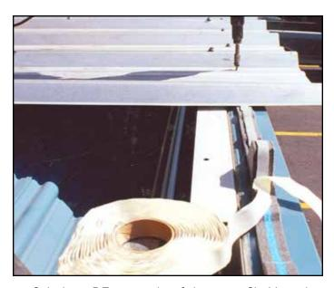
o. Galvalume R-Type panel roof sheets are 3' wide and attach to the structure using Zac head screws for secure placement.
