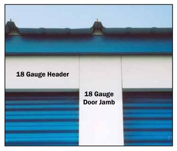
a. Door jambs and headers are constructed of prefinished 18 gauge material, which is 2-1/2 times thicker than the industry standard 26 gauge material. Jambs and headers feature no exterior fasteners giving a clean, finished look.
