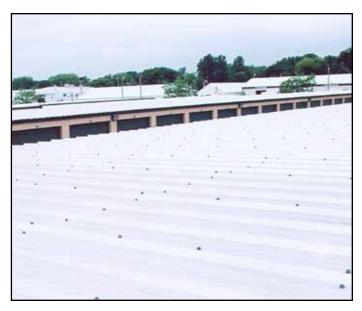
o. An installed galvalume R-Type panel roof with exposed fasteners.
