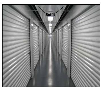
x. A soffit ceiling is recommended if using door alarms. This gives access to the alarms for maintenance purposes. Trachte can supply a 2-T8 bulb lighting package which is recommended.
