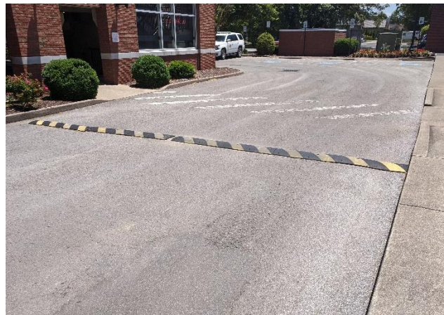
Speed bumps are not an approved traffic calming technique for residential streets.
