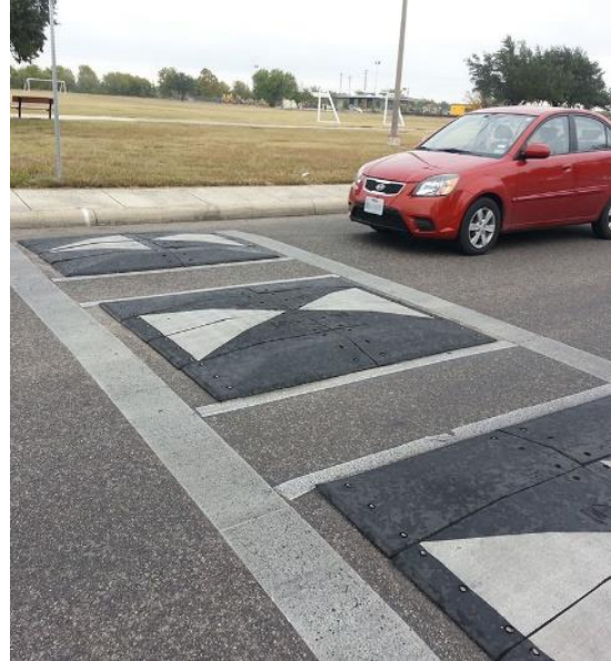
EXAMPLE: Speed cushions that may be permitted in the City of Alabaster.
