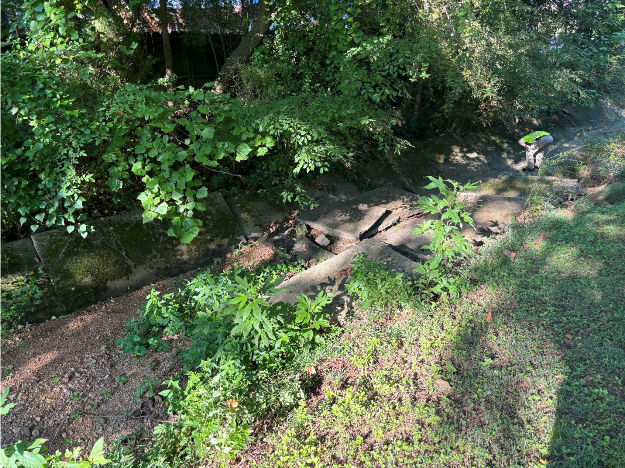
concrete flume repair on independence drive 07-22-2024
