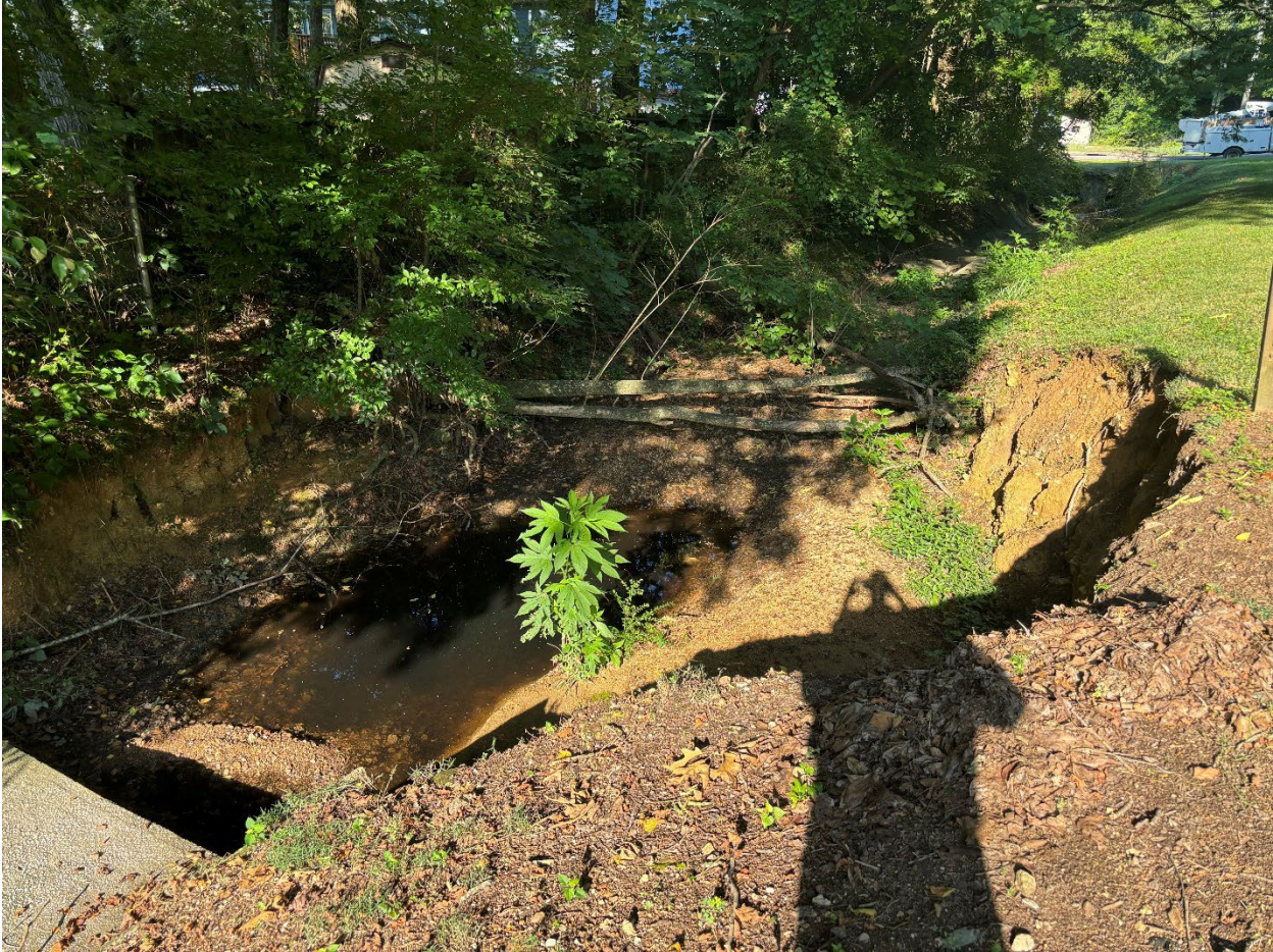
concrete flume repair on independence drive 07-22-2024
