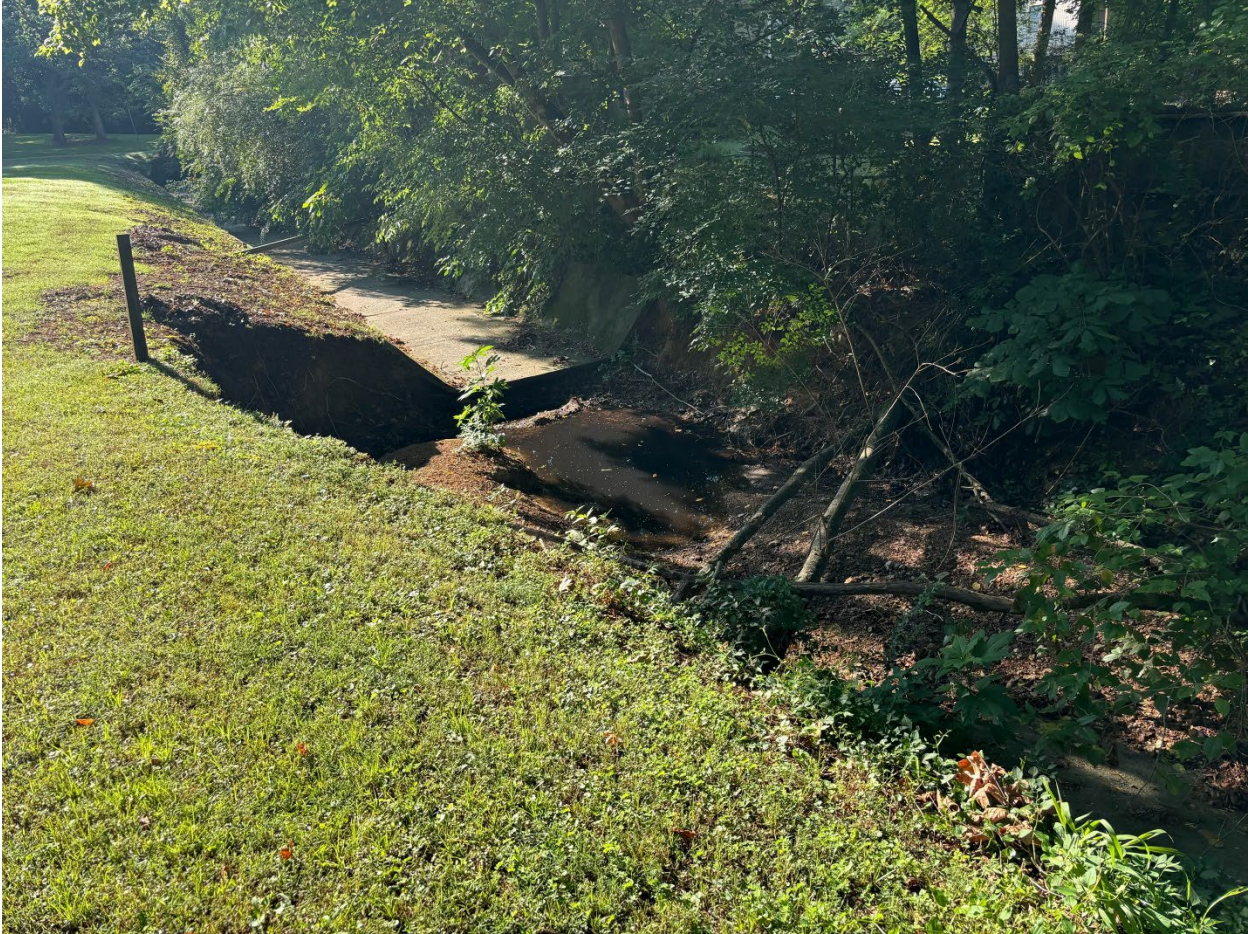
concrete flume repair on independence drive 07-22-2024
